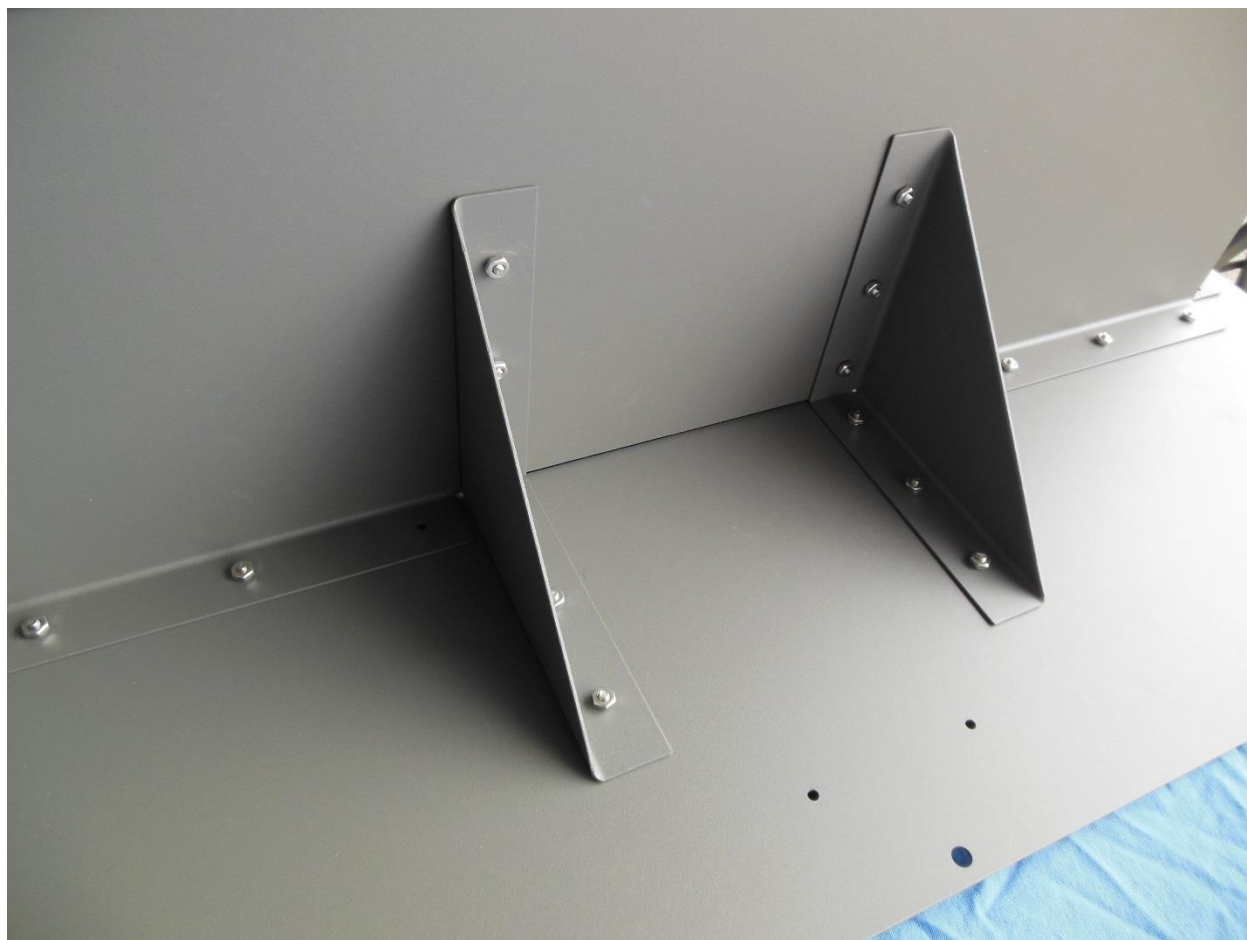
Figure 6. Hat Shelf – Braces as installed.
