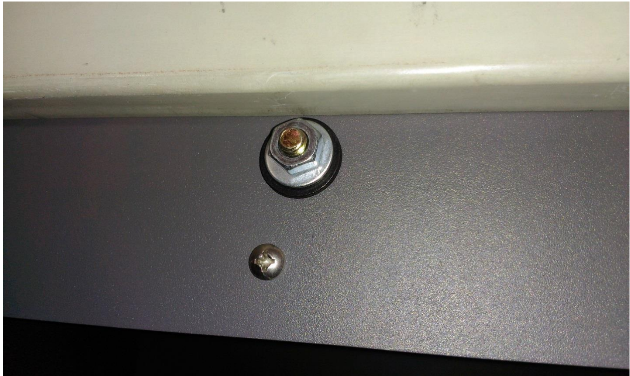
Figure 13. Finished mounting bolt installation.
