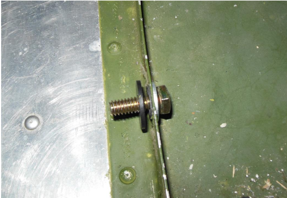
Figure 11. Mounting bolt showing washer, e-clip, and first neoprene washer.
